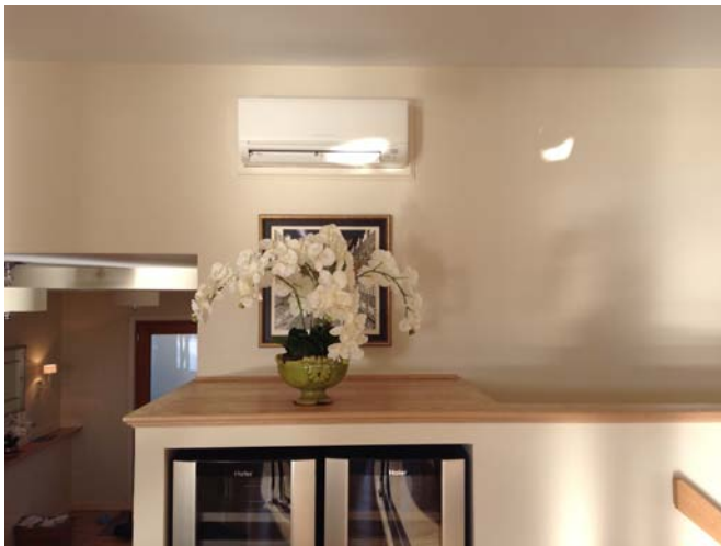
Picture above: Picture of wall hung interior unit
