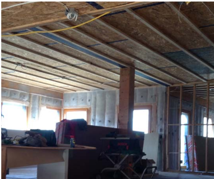
Picture above: Taped air tight layer of interior OSB roof sheathing.
