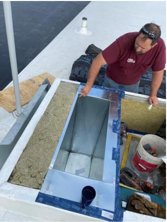
Lining the inside of the ERV curb with layers of 2" Rockwool board and filling the space around the ducts with Rockwool batts
