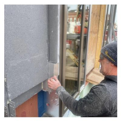
Installation of cladding clips and insulation
