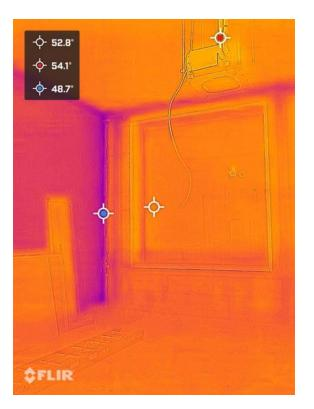
Third floor, NE corner, prior to adding more interior insulation to mitigate thermal bridge at building intersection with neighbor.
