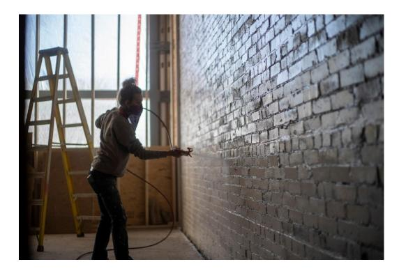
Applying the first coat of Visconn on masonry walls, second floor, typical.
