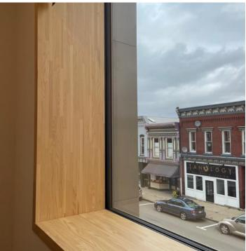
Detail of extended curtainwall frame
