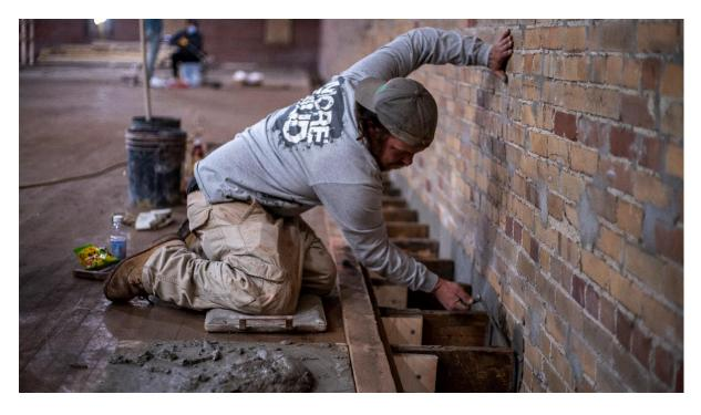
Parging at joist pockets before Visconn application, typical.
