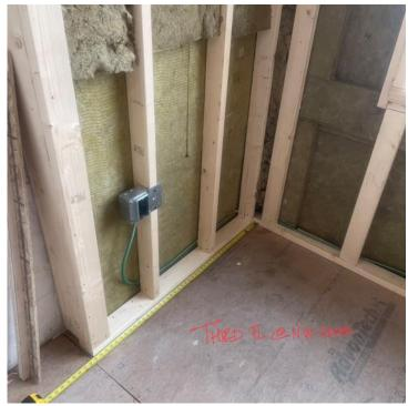
After addition of return wall to insulate corner
