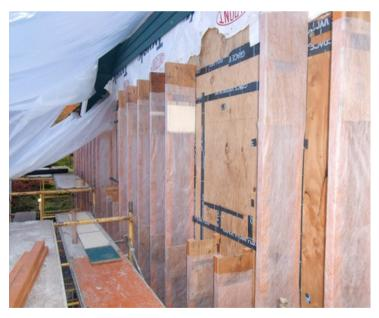
We cut air leakage through our house by over 80% by careful sealing of existing exterior wall plywood sheathing, ceiling sheetrock, and ground floor plywood floor to induced 0.75 ACH @ 50 Pa.
