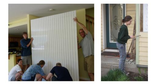
We reinsulated our ground floor to R50 and added insulation to the inside and outside of our concrete foundations to reduce the thermal bridge through the foundations.
