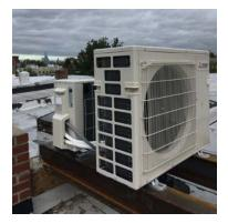
Because of the need for mechanical cooling and dehumidifcation in summer in New York, ducted heat pumps were selected to supply cooling and dehumidifcation in summer as well as heating in winter. The ducted indoor units require relatively little space and provide zoned controls for the owners.
