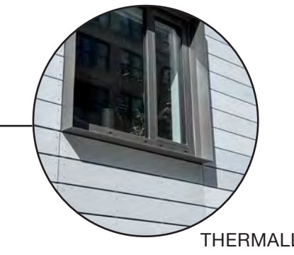
THERMALLY BROKEN EXTERNAL SHADING ELEMENTS
