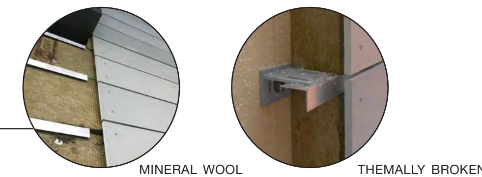
MINERAL WOOL & VENTILATED RAINSCREEN SYSTEM
